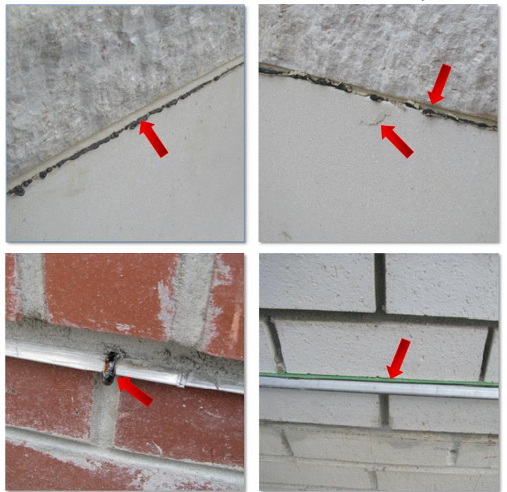
The membrane needs to be protected from UV rays & due to the sun and heat, the membrane will flow to the front face and potentially damage the masonry & mortar...and be unsightly.
